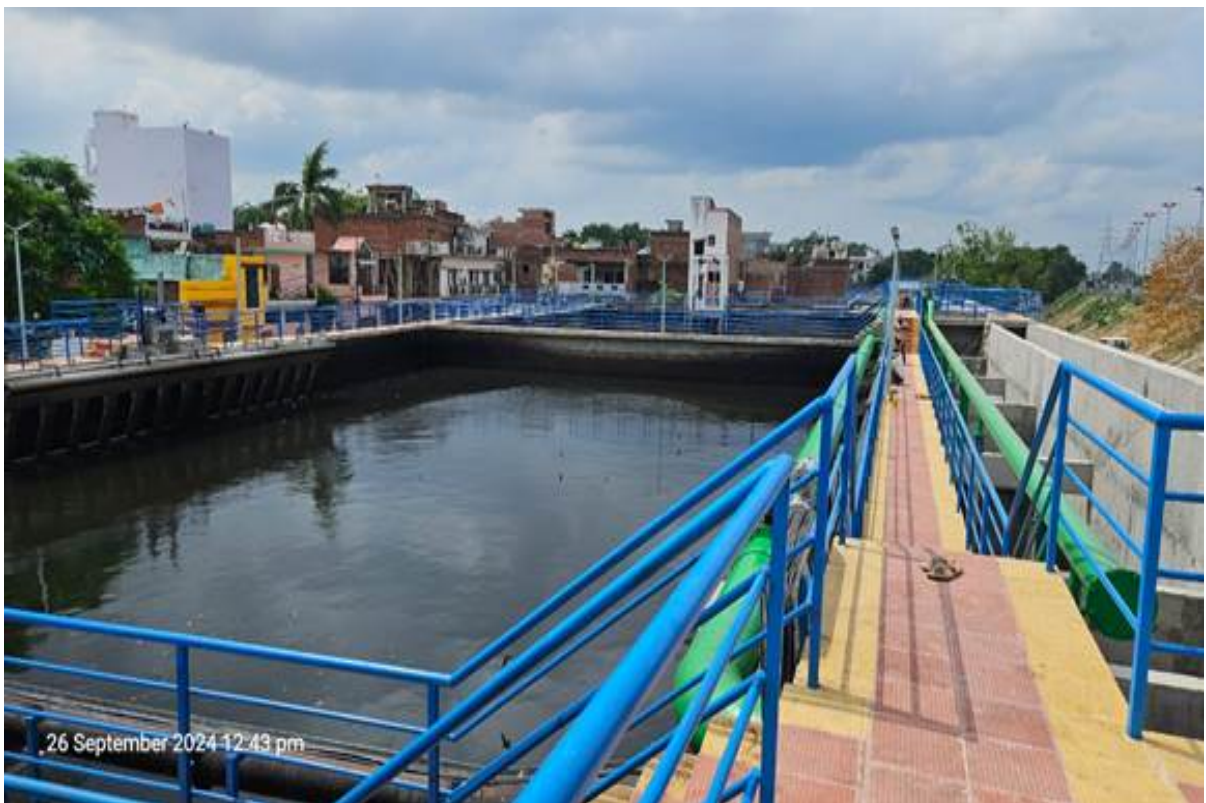
39 MLD STP at Lucknow
